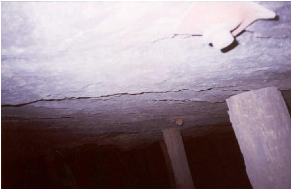
**Figure 5.3.5** *Roofbolt installation in main training site after training of team leader. Support at correct angle.*
