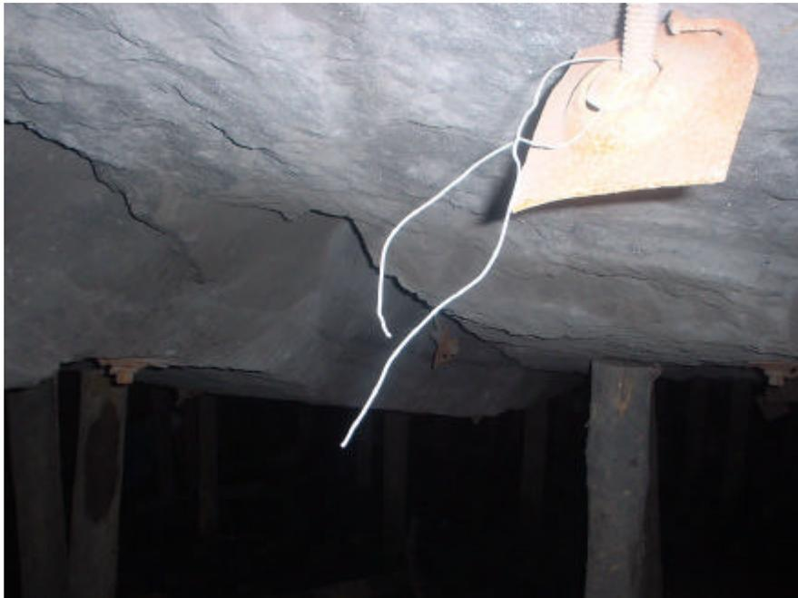
**Figure 5.3.11** *Roofbolts installed next to a fault plane*
