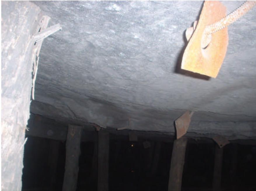
**Figure 5.3.10** *Loose roofbolts in the back area of the control stope*
