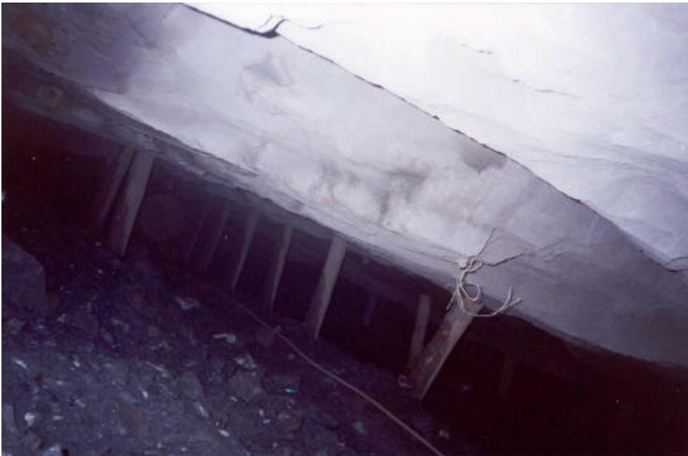
**Figure 5.3.7** *Conditions in the face area before replacement team leader took over. Minor FOG resulting in the development of a brow.*
