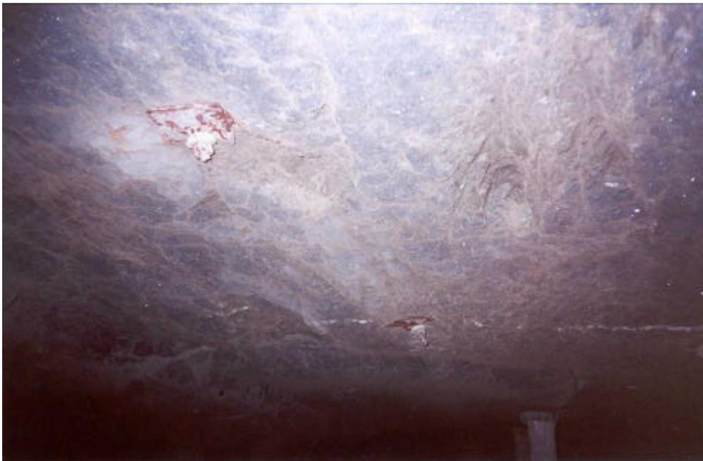
**Figure 5.3.3** *Roofbolt installation in main training site before training of team leader. Shows bolt angle incorrect and not correctly seated.*
