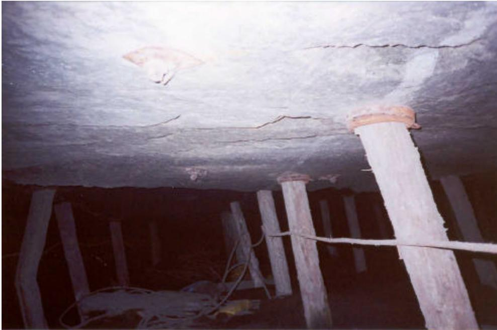
**Figure 5.3.4** *Support installation in main training site before training of team leader. Shows installation of mine pole as incorrect.*
