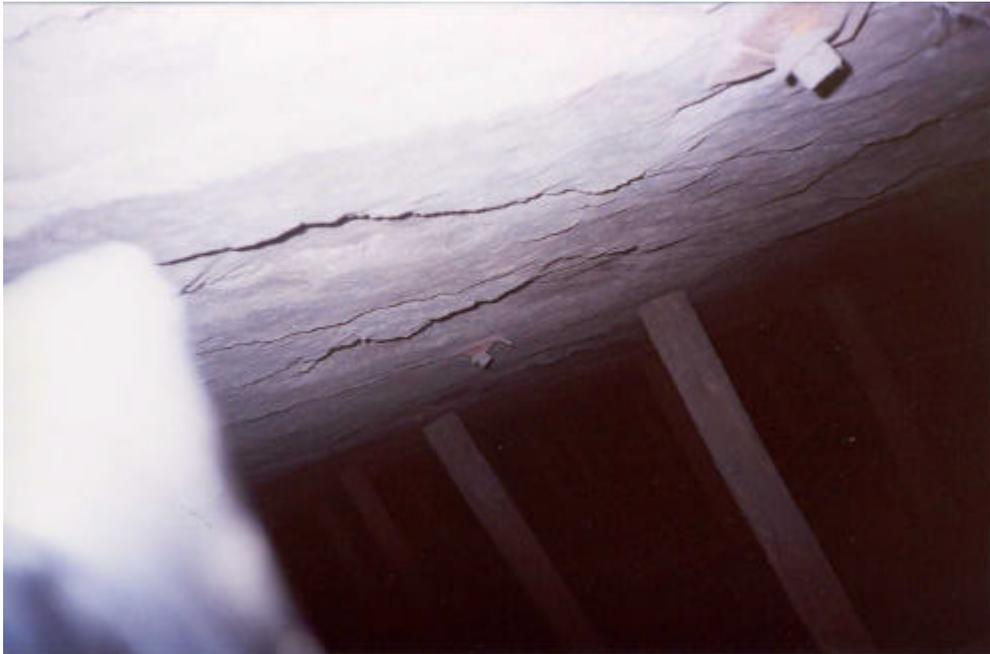
**Figure 5.3.6** *Support installation in main training site after training of team leader. Shows improved bolt angle to dip of hangingwall.*
