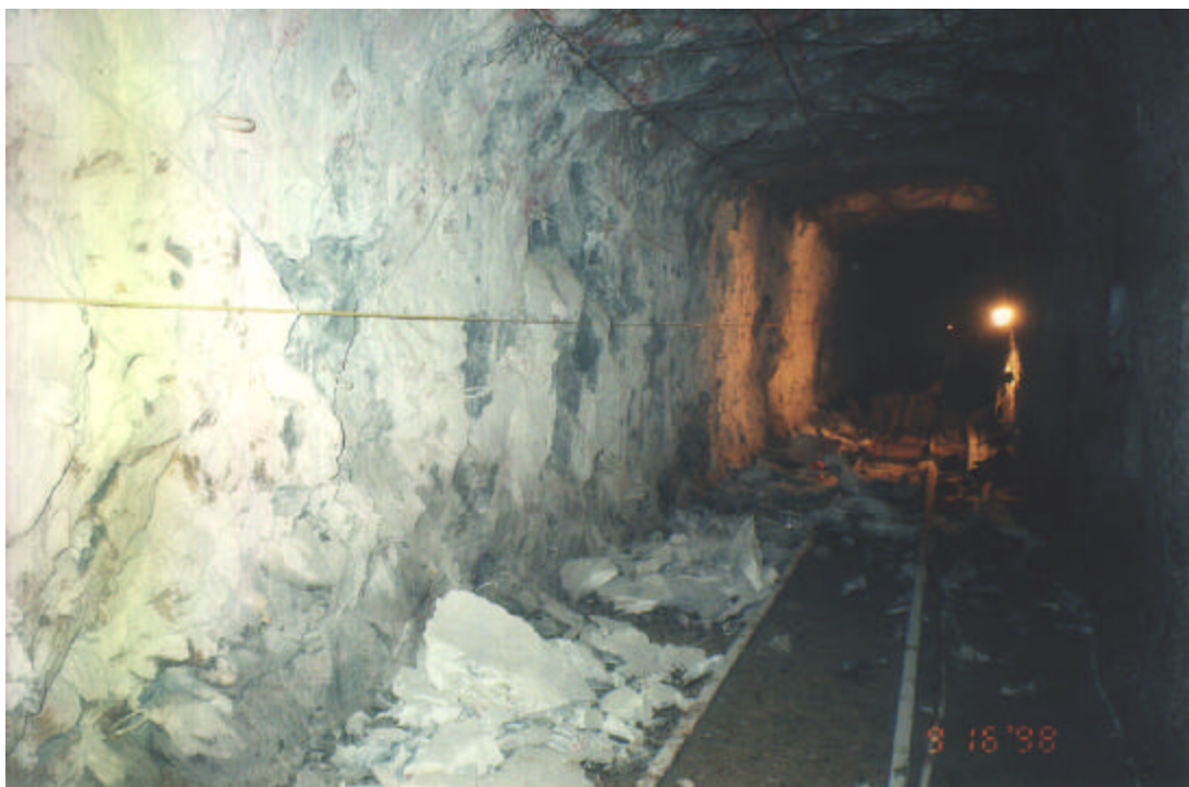
Figure 4.7.14 Photograph showing rockburst damage along the experimental tunnel. The area of high intensity damage is in the foreground and low intensity damage towards the background (after Le Bron et al., 1999).
