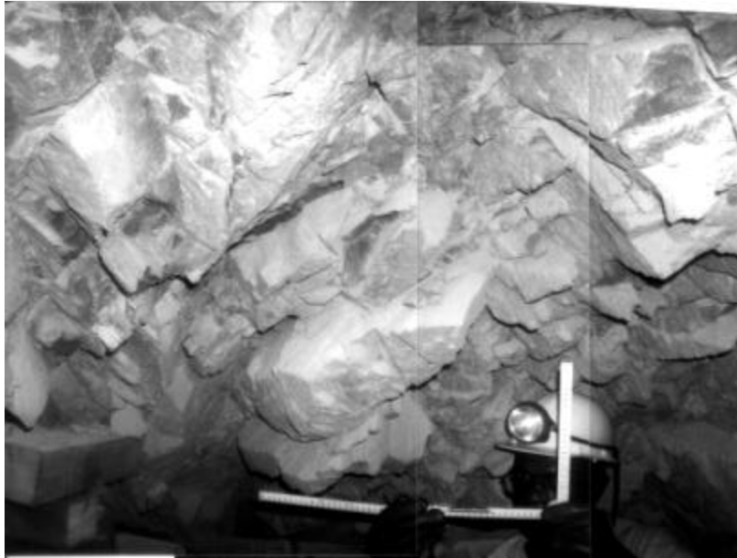
Figure 4.8.10 Example of a blocky hangingwall.
