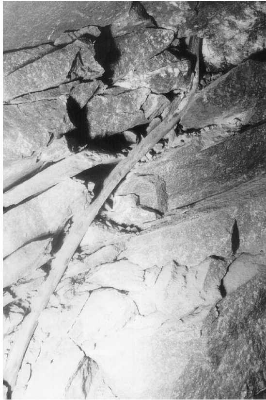
Figure 4.2.11 Shear deformation of smooth bar rockbolt.
