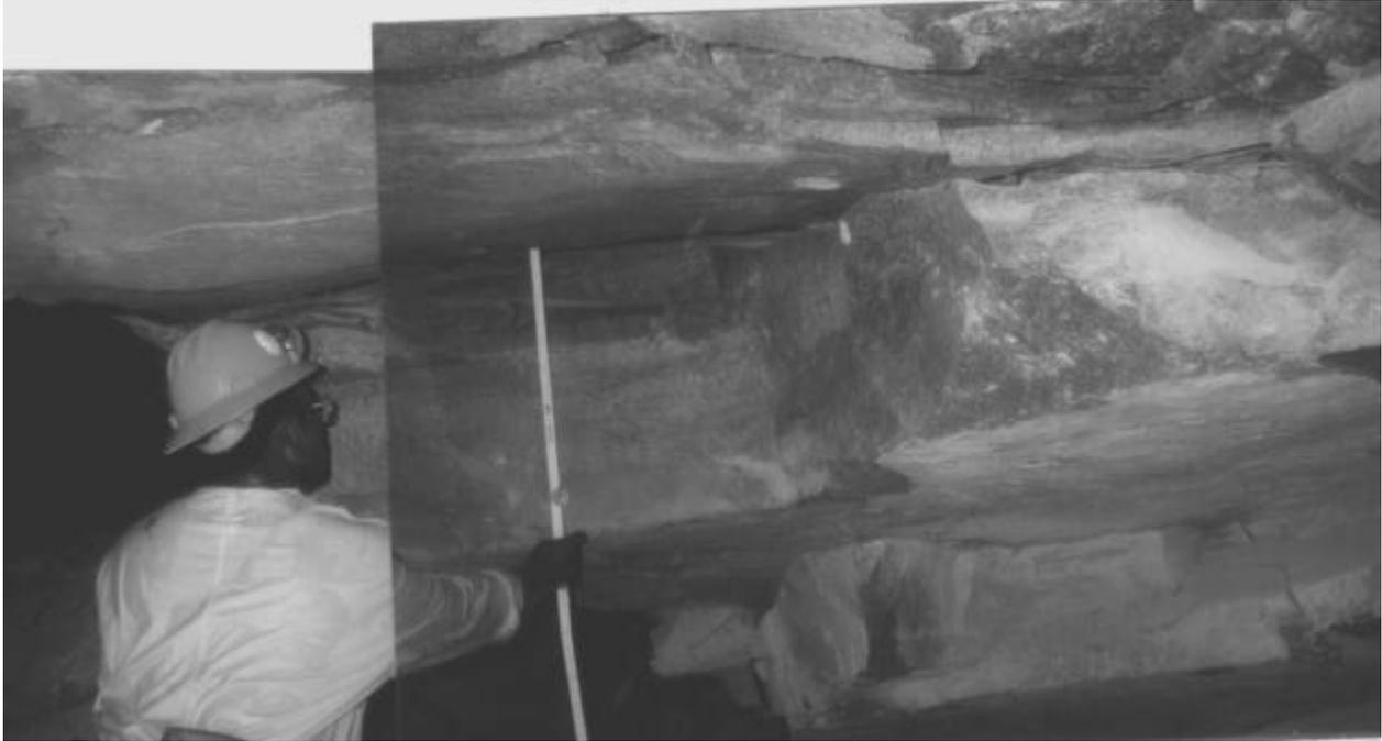
**Figure 3.3.5** *Fallout along a shaly bedding plane (face to the right).*
