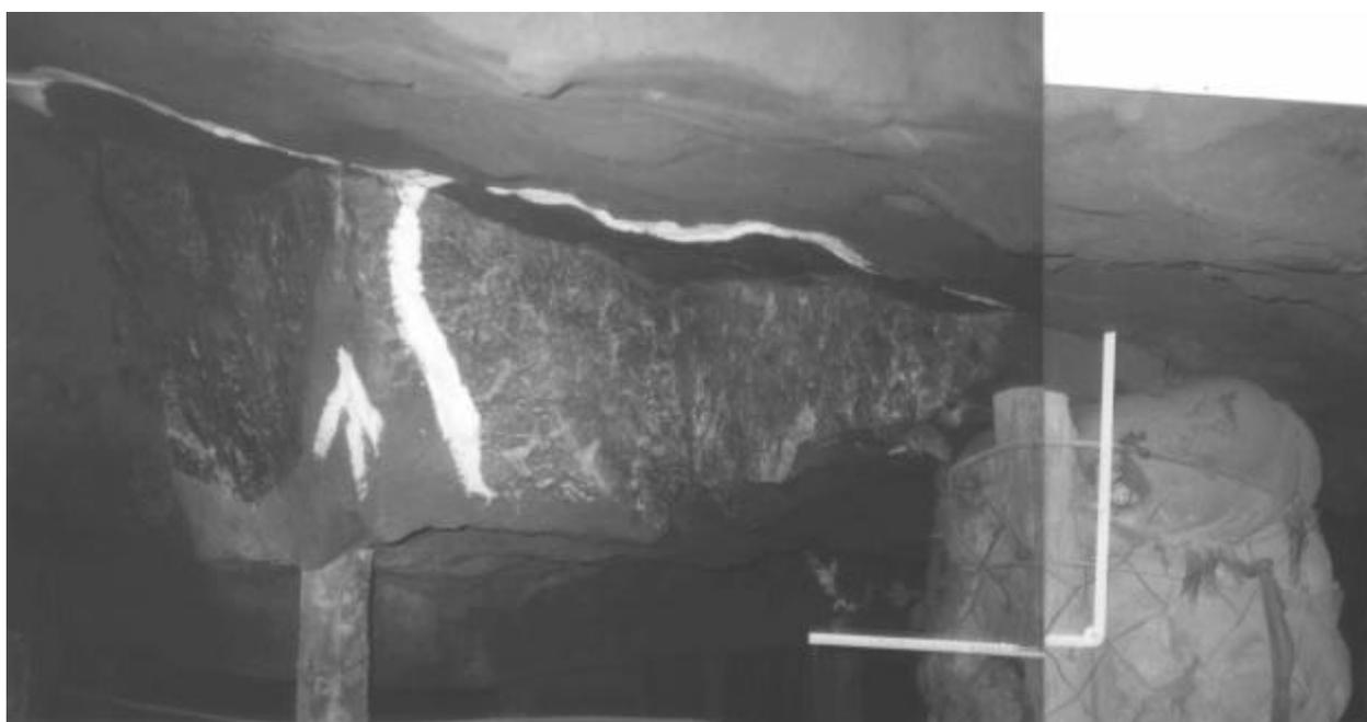
***Figure 3.3.7 The effect of reef parallel and reef perpendicular structures on the hangingwall conditions.***
