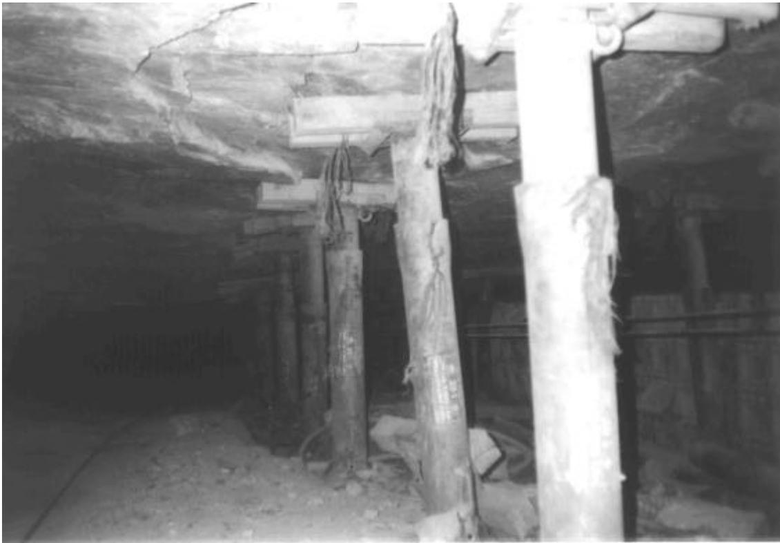
**Figure 3.3.3 Strong hangingwall – siliceous quartzite (face to the right).**
