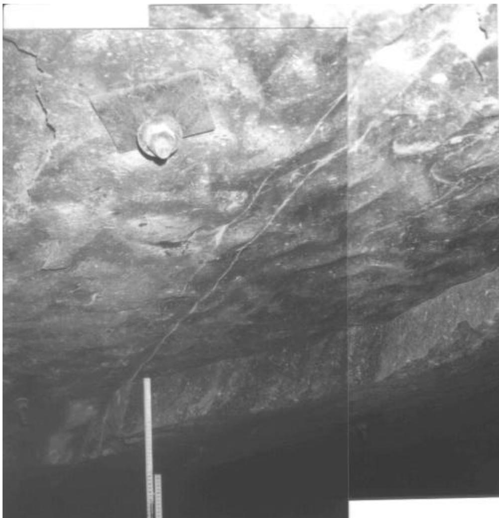
**Figure 3.3.4 Ripple-marked bedding plane defining fallout (face to the right).**
