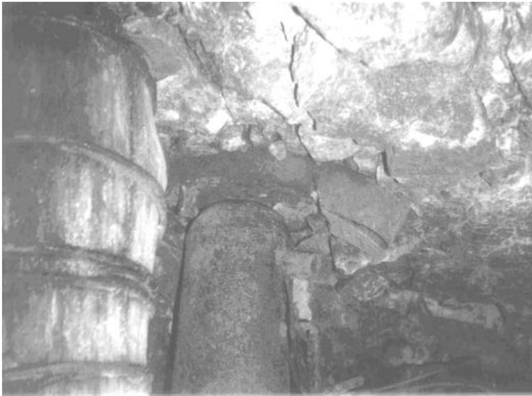
***Figure 3.3.1 Punching of support unit into weak, argillaceous hangingwall (face to the right).***
