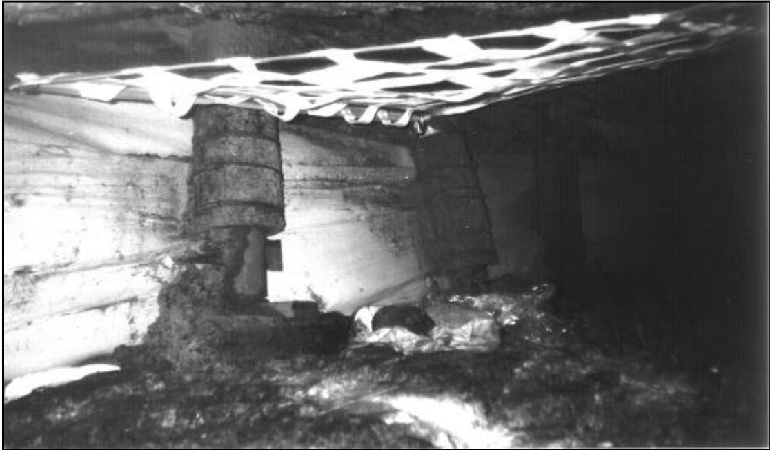
**Figure 3.7.17**      *Net pulled tight by hand only.*
