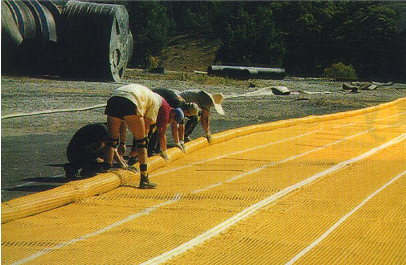
**Figure 3.7.22**      *Rolling up the mesh on surface at Springvale colliery.*
