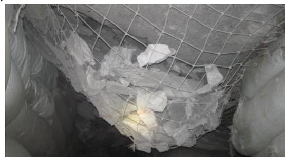
**Figure 1. Net retaining broken hanging without rock bolts (in-stope steel rope netting without tendons, Deep level mining in high stress)**
